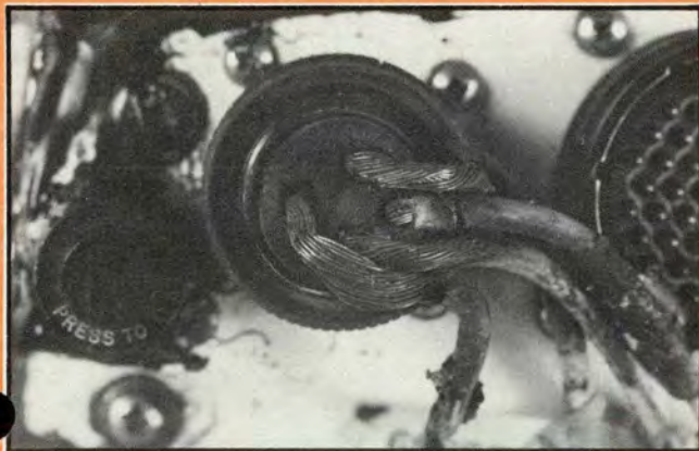
This is a typical example of the wiring damage resulting from a water/glycol fire.
